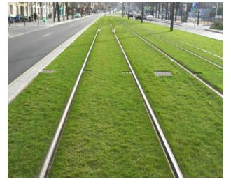
In some locations there is no choice of track type. For example, the tracks must be embedded where other vehicles will operate on or cross the tracks. In other areas the track type is being evaluated based on operations, maintenance, cost, and aesthetics.
